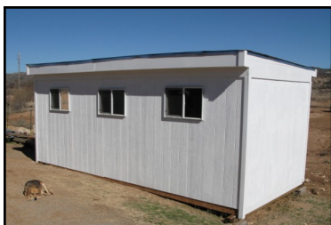
The "Hoppy Shack" near its completion
